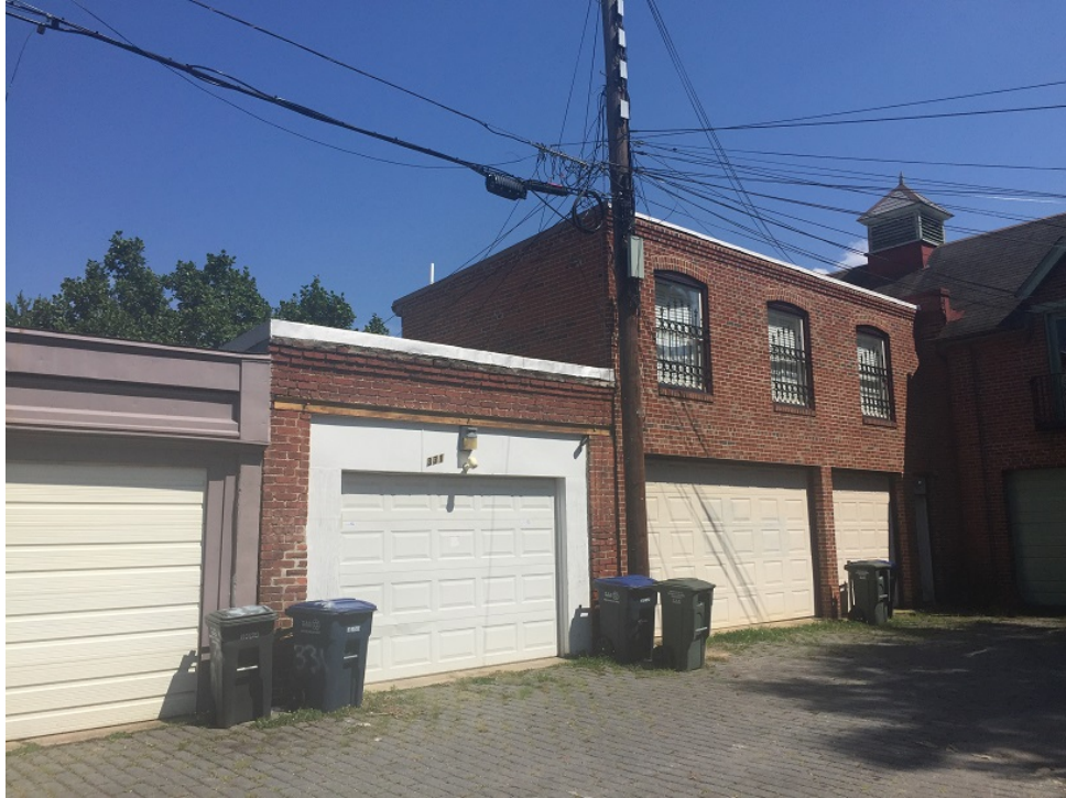
VIEW FROM ALLEY- LOOKING EAST
