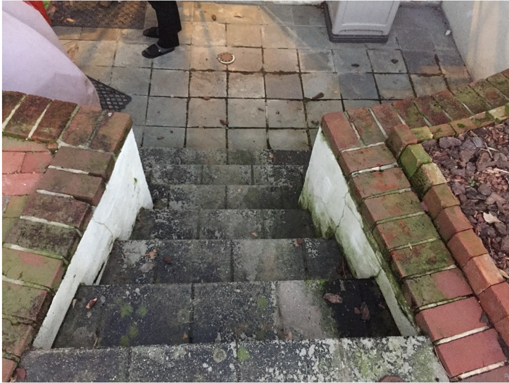
EXISTING AREAWAY & STEPS TO GRADE
